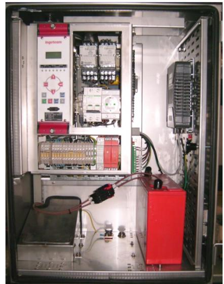
All equipment in the cabinet are easily removable for repair / replacement. The battery has an industrial connector that allows quick replacement. The cabinet has a removable tray to install telecommunications equipment and allow proper configuration and maintenance.
